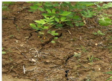
(b) 墙脚外裂缝
