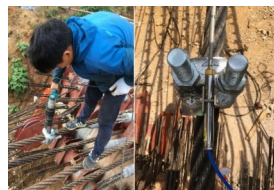
(a) 绳扣和高精度位移计布置
