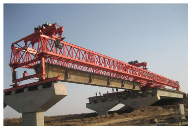
(c) 架桥机安装T梁
